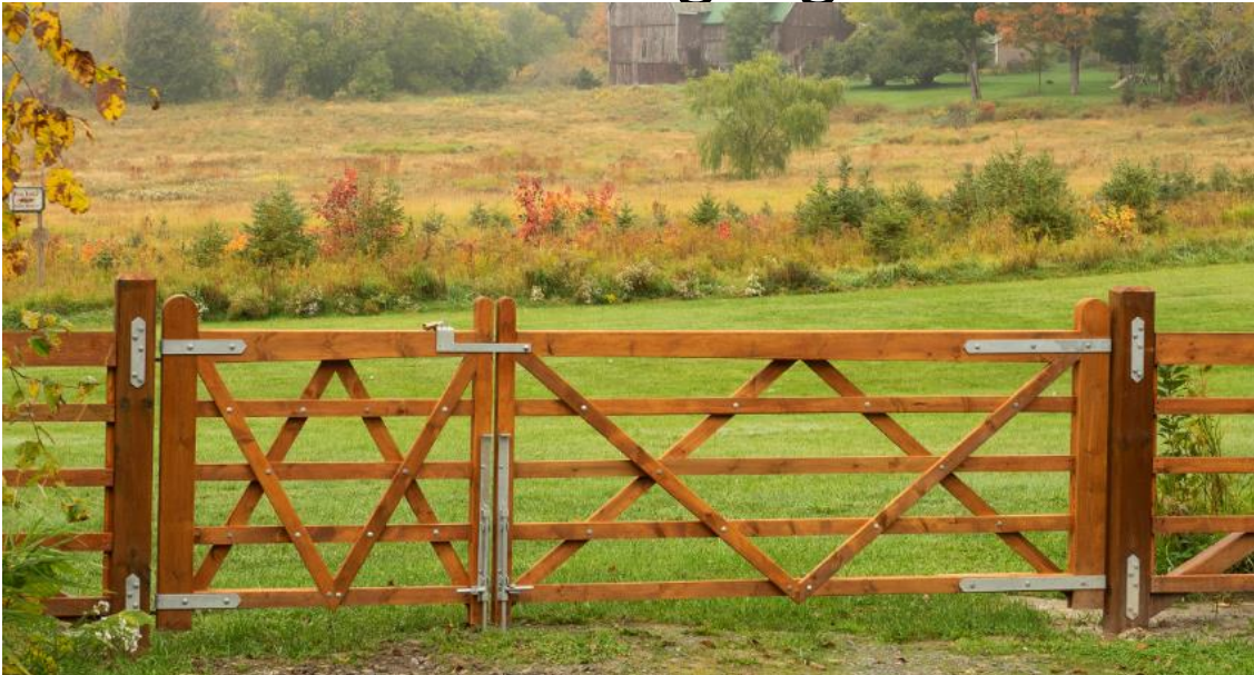
New Gate and Signage
